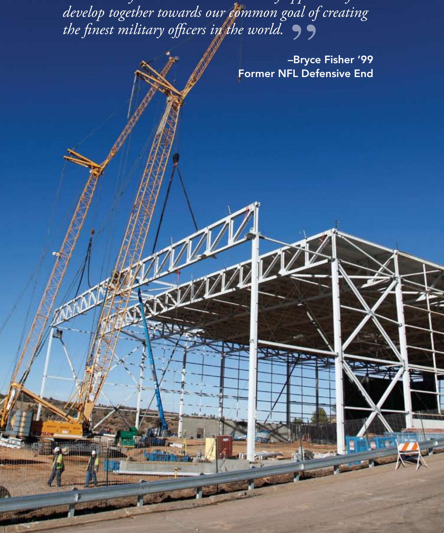
Holaday Athletic Center construction
